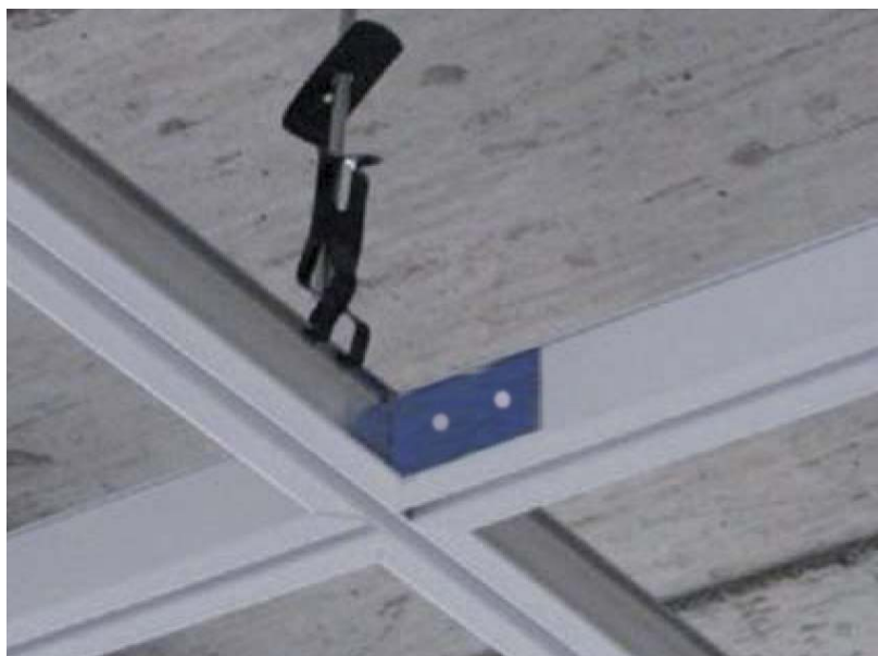
Clean mitred cross runner intersection.
