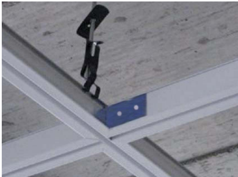
Clean mitred cross runner intersection.
