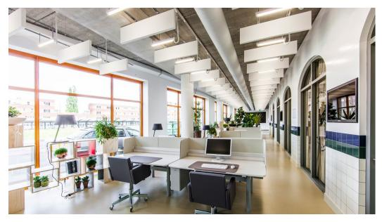
Rockfon Contour Baffles are frameless, vertically-hung acoustic panel with very-high acoustic absorption properties. Baffles can be hung in random patterns at varying heights, or in a more traditional linear configuration to assist with both the absorption and diffusion of sound. They are ideal for restaurants and cafes where acoustics are compromised by surrounding hard surfaces. Rockfon Contour Baffles are an economical and easy to install solution to improving the acoustics in any space.
