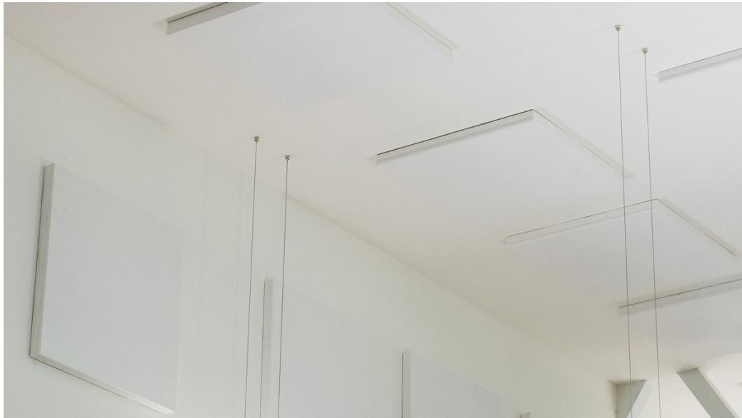
Rockfon Sonar Activity panels assist in reducing reverberation in high-activity areas using a 'direct-fix' solution to minimise any loss of ceiling height. Ideal for retrofitting onto hard surfaces such as plasterboard and concrete whilst maintaining an attractive aesthetic. Sonar Activity panels maintain high-NRC values despite the direct-fix installation method. They are ideal for cafes and restaurants, retail environments and other loud spaces where installing T-grid ceilings is impractical.
