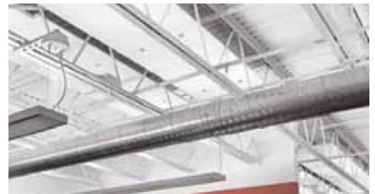
OPTRA Capz, installed 165mm from a metal deck.
